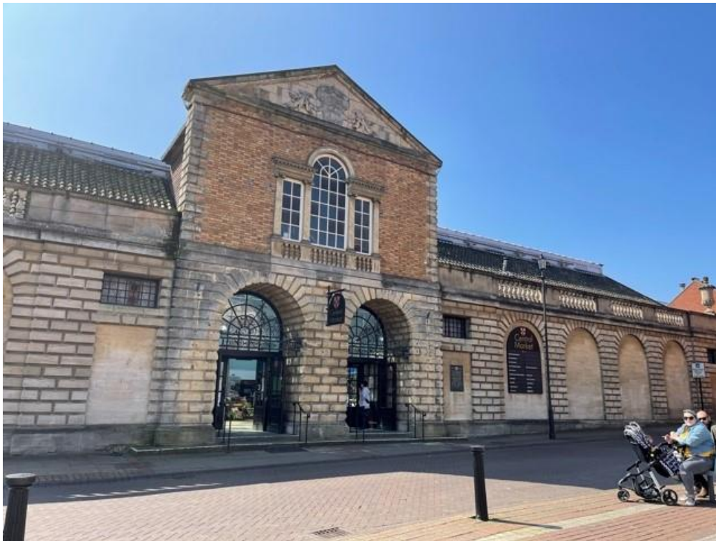
Existing North facing elevations to City Square. Blind arcade evident
