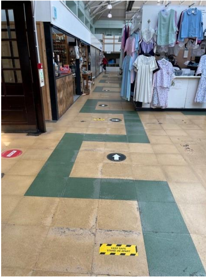
Existing Terrazzo floor within the main Central Market building
